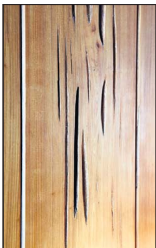
Detail of the pecky cyprus paneling, with long cavities caused by a fungus.
